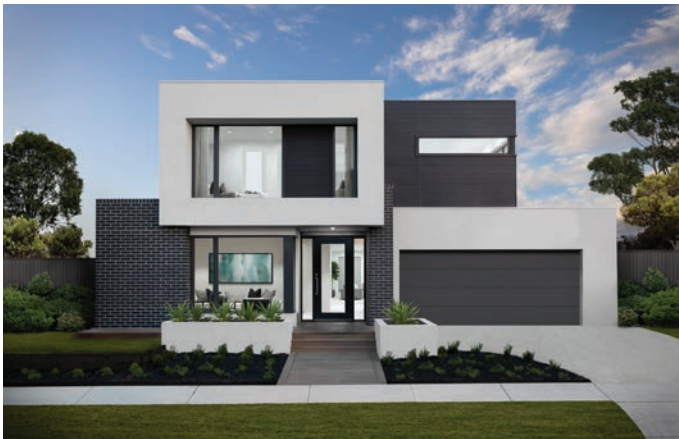
Flat Roof - Boutique Homes (Grange)
