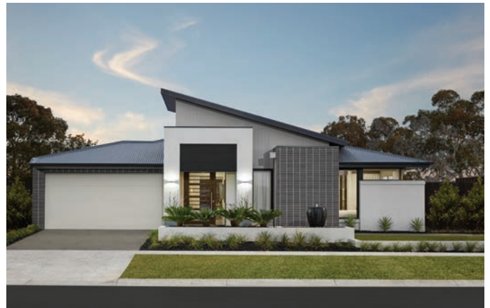
Skillion Roof - Metricon Homes (Botanica)
