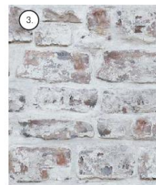
ORIGINAL WHITE PAINTED BRICK, WATER JET BLASTED TO REVEAL BRICK
