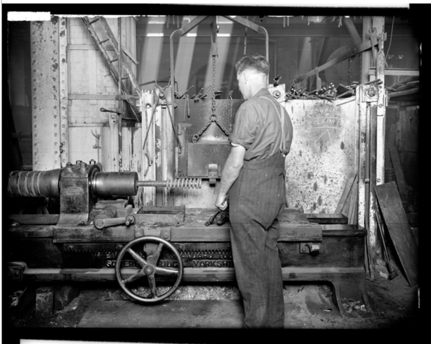
Forming a coil spring on the Witham Spring Coiler, c.1920s. (Ref: NSW State Records B281357)
