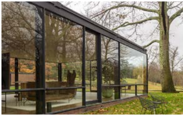
1. CLEAR GLAZED NEW OPENINGS, MINIMAL FRAMING
