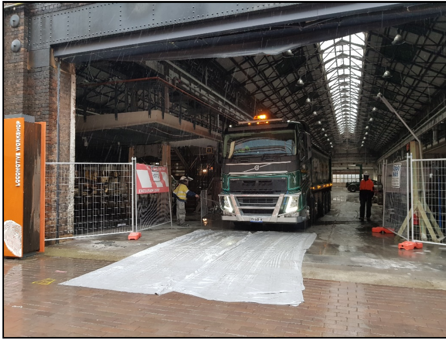
Photo 3: Vehicle wheel wash.
