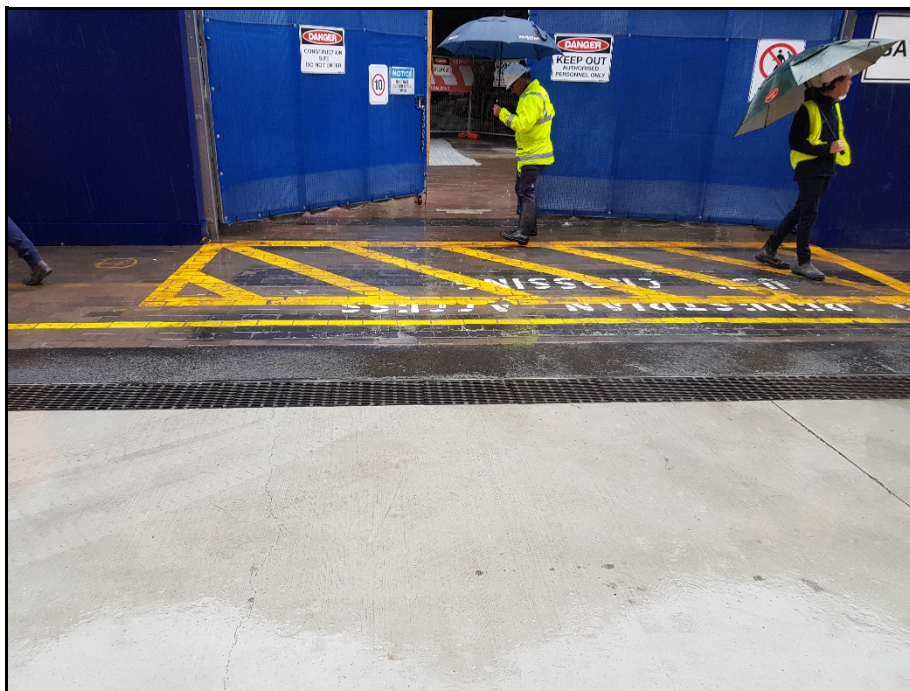
Photo 4: Stormwater drain along Locomotive Street outside vehicle wheel wash area.
