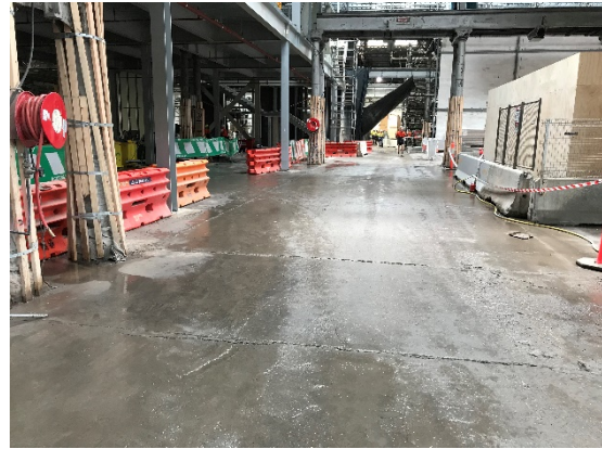
Photograph 2: Concrete hardstand/physical barrier across along the central spine of Bays 1 – 4A
