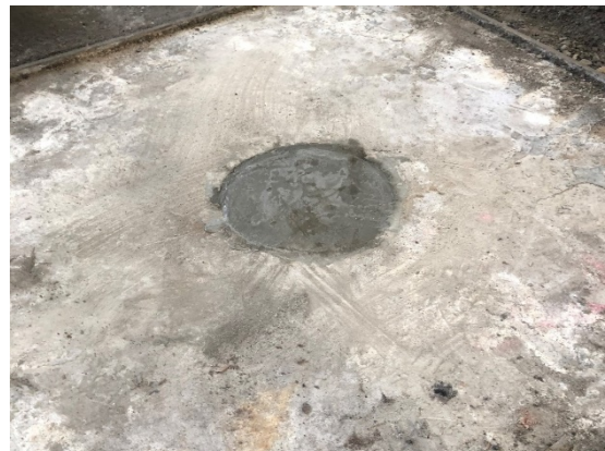
Photograph 4: Intrusive boreholes/concrete hardstand reinstated following sampling works.
