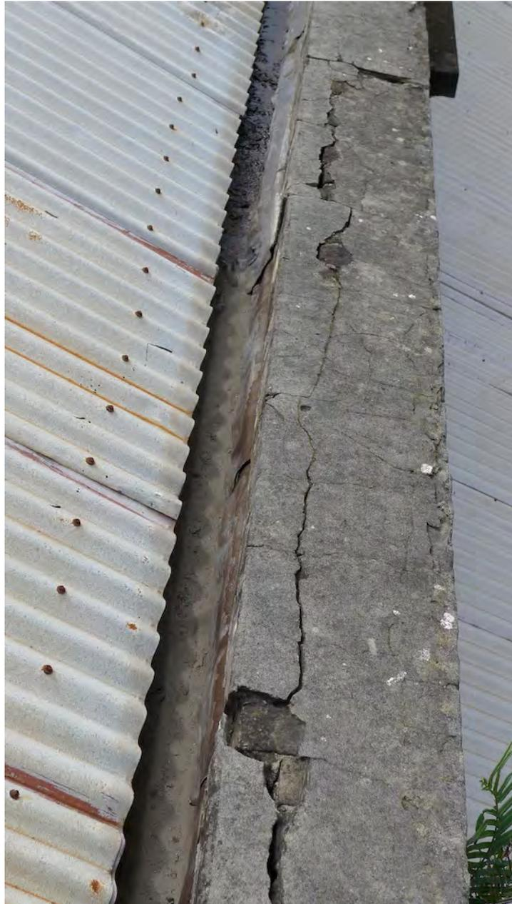
Figure 11 – Note that the breakdown of the render is uncovering underlying fractures of the sandstone coping.
