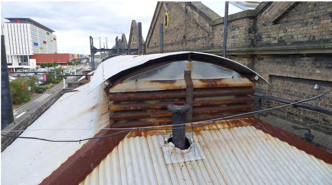
Figure 13 – The roof covering of the Bay 2 Annex. Note the rusting hip flashings, the damaged and corroded louvers, the distorted capping to the surmount and poorly flashed penetrations.
