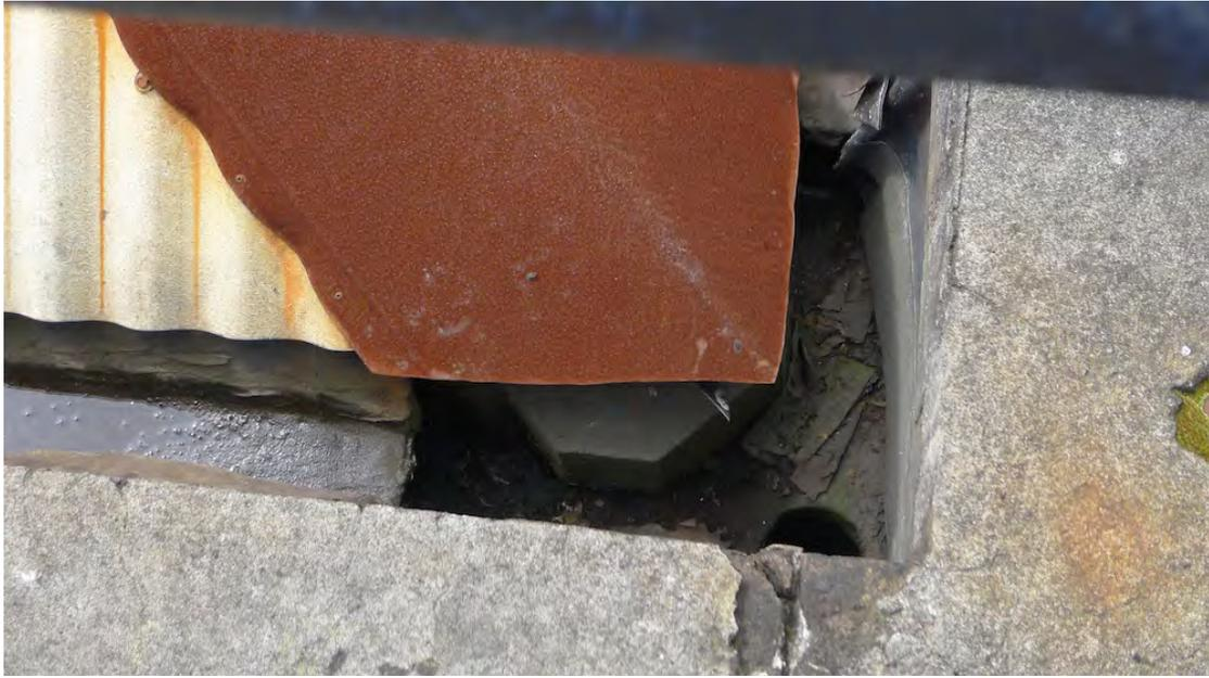
Figure 14 – Detailed photograph of the guttering of the Bay 2 Annex. Note the downpipe appears to discharge into a concealed downpipe. The associated plant growth would suggest the drainage line no longer functions and the surface water saturates the masonry.
