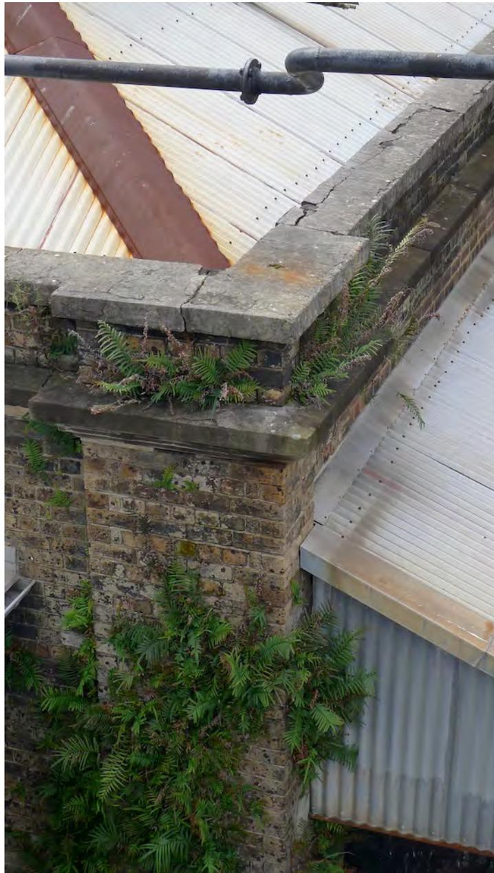
Figure 10 – Corner of the Bay 2 Annex showing plant growth indicating chronic saturation probably caused by the breakdown of the drainage within the pier. This occurs in the southeast and southwest corners.
