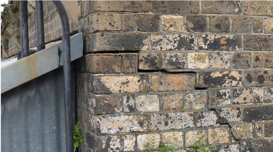
Figure 8 – Cracking of the brickwork caused by rust jacking.
