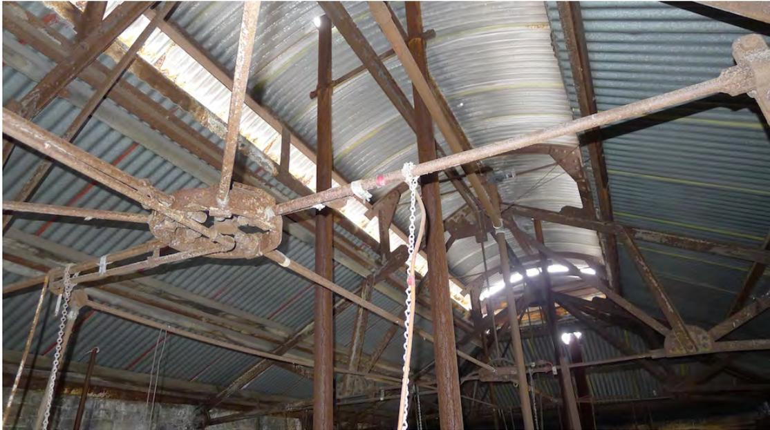
Figure 12 – Internal view of the roof structure of the Bay 2 Annex. Note the complex junction of tie rods at the hip apex.
