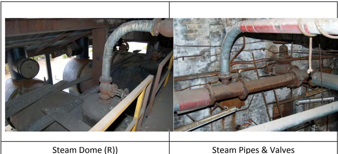
Each boiler is fitted with safety valves, which are designed to release excess steam to the atmosphere in the event that pressure within the boiler exceeds a set limit. The steam pressure is measured with gauges. The safety valves are located on top of the boiler.
