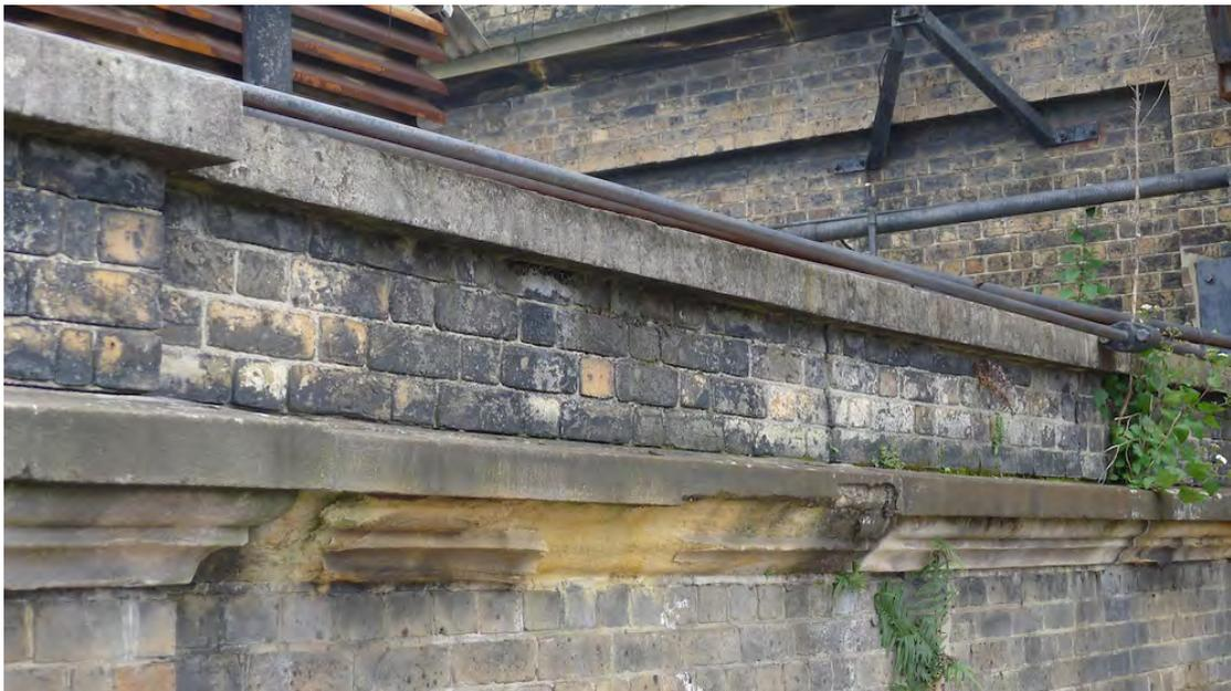
Figure 9 – Erosion of sandstone elements and plant growth on the Bay 2 Annex.
