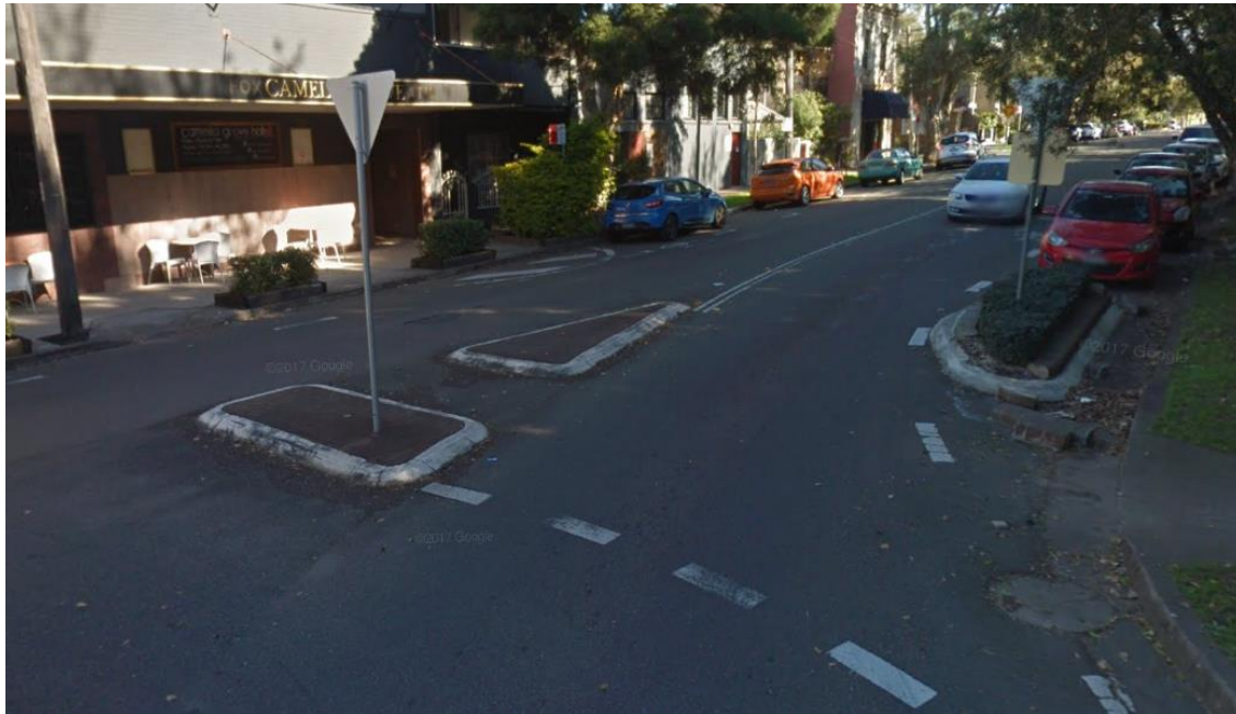
Figure 2.8: Refuge Island and Pedestrian Infrastructure at Roundabout (along Henderson Road)
