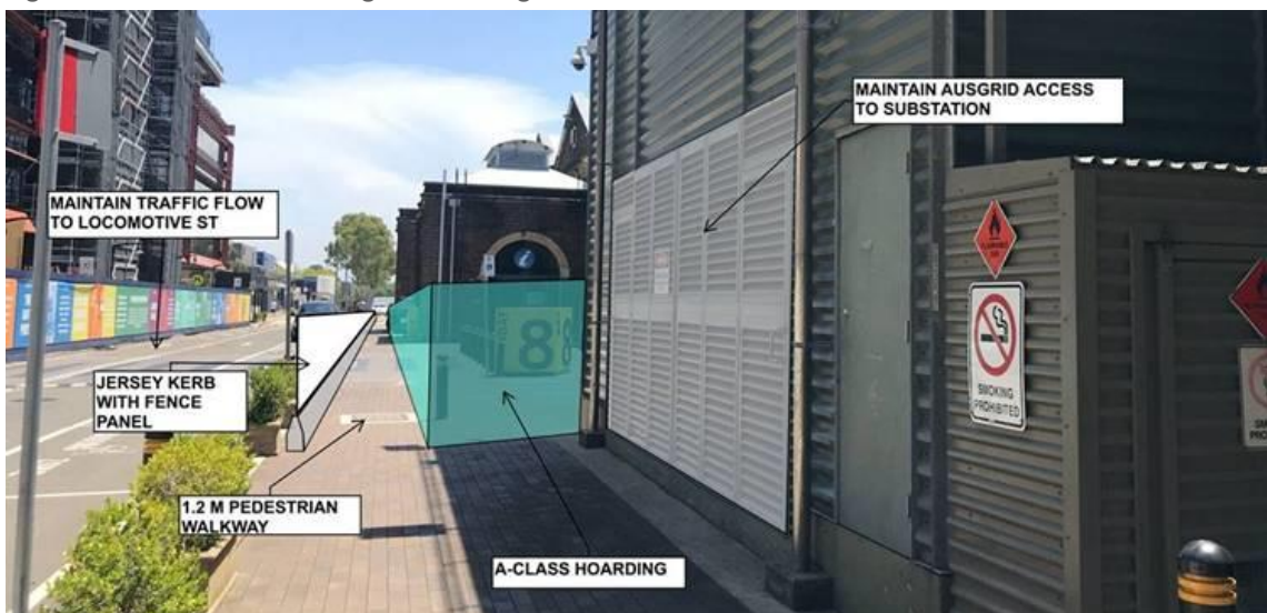
Figure 3.4: Pedestrian management along Locomotive Street
